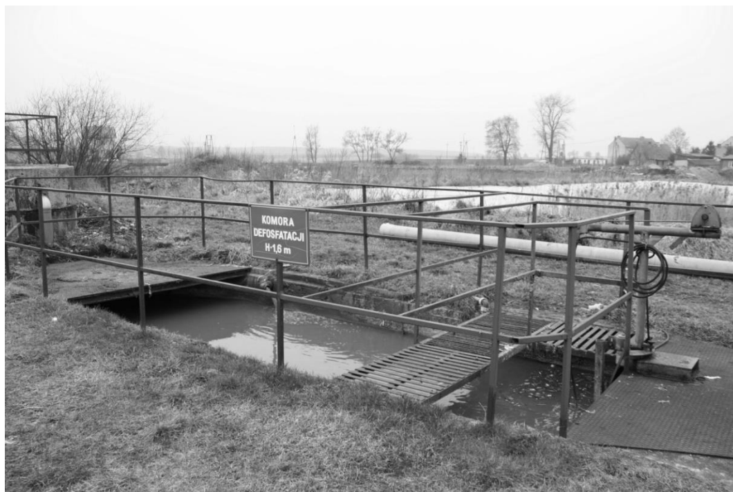
Figure 1. Anaerobic chamber
