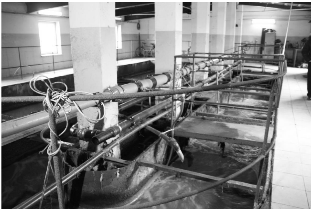
Figure 3. Second aerobic chamber
