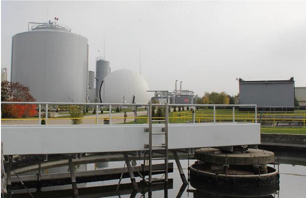
Fig 3. Fermentation chamber and biogas storage
