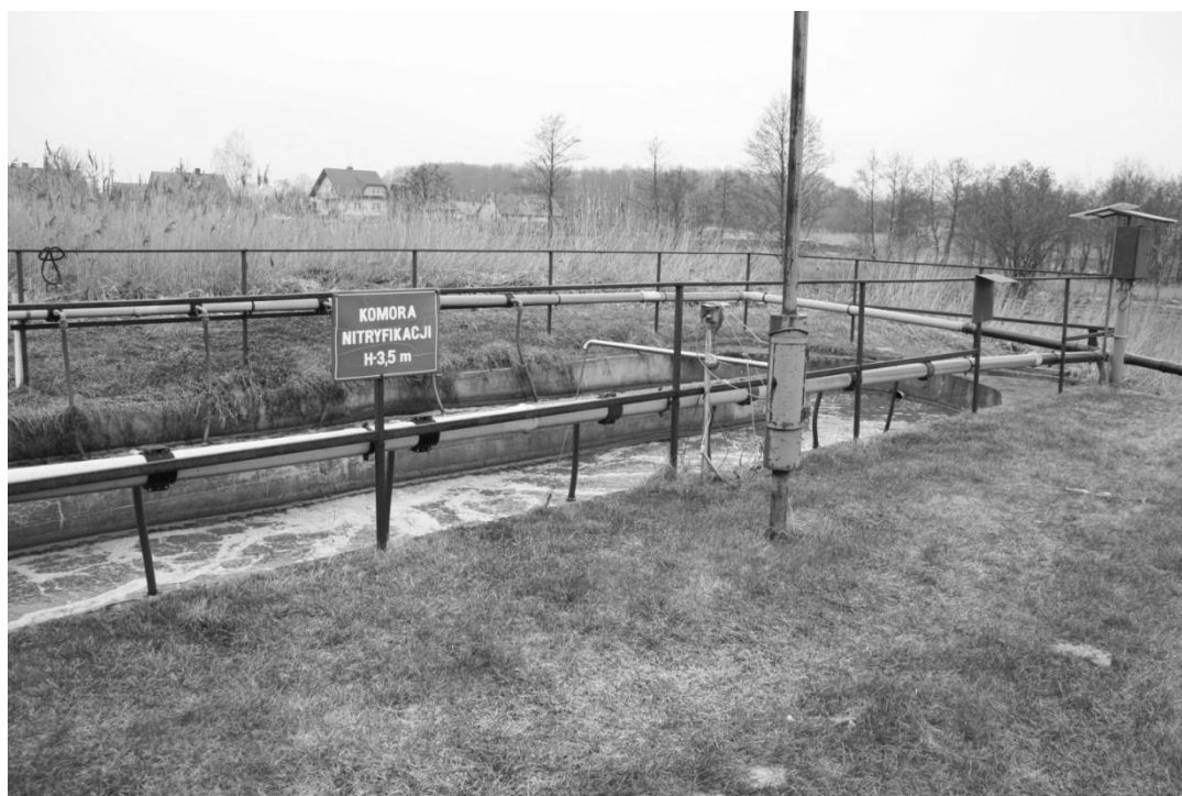
Figure 2. First aerobic chamber
