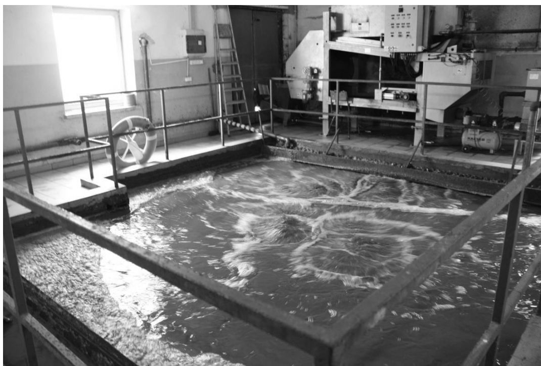
Figure 4. Sludge stabilization chamber
