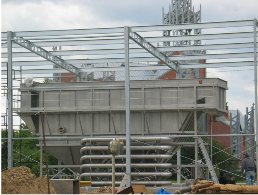
Fig. 4 Flotation unit during modernization.
